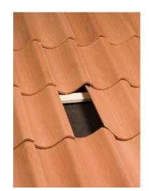
**ENG:** Remove one tile to which you will install a Universal tile pass-through. Make sure there is not a roof truss at that spot.
