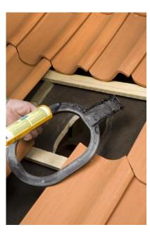
**ENG:** Put rubberized bitumen sealant on the bottom surface of the underlay seal, if the underlay seal is made of bitumen.
