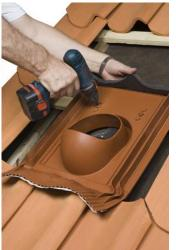
**ENG:** Mount the top part of the pass-through onto the batten with two short screws. Choose an appropriate seal of the three seal alternatives for the top edge of the pass-through. Remove the protective film of the tape from the pass-through, and mount the seal onto it. Make sure that it is in the correct location sideways.
